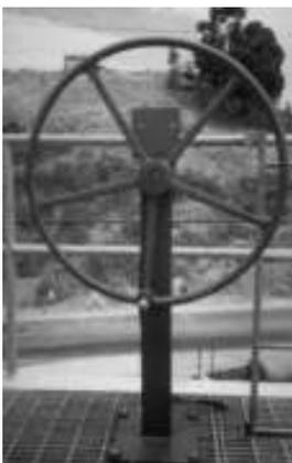
The hydraulic extension for gear operators is essentially a hydrostatic transmission.
