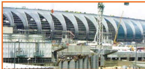
Expansion project - Dubai Airport, UAE
