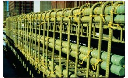
Rebar coated with 3M™ Scotchkote™ 413. 17
